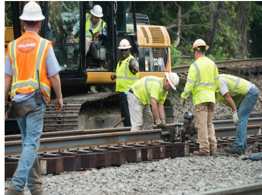
Crews complete track construction activities
