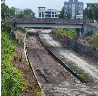
NCDOT rail corridor near 3 rd Street in Downtown Wilmington
