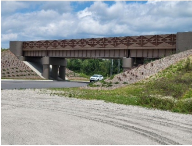
New railroad bridge near Lumberton, NC
