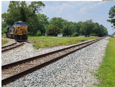
Wye connection in Warsaw, NC
